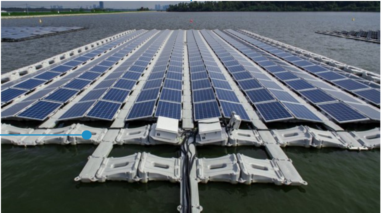
Floating solar panels installation
